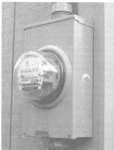
Fig. 8-7 Typical outdoor weatherproof kilowatt-hour meter and its socket.
