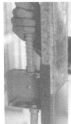
Fig. 12-7 This shows the corrugations on ENT, which allow it to be bent by hand (a “pliable” raceway according to the NEC definition). A snap-on connector has been added, which will lock in place when it goes into one of the knockouts in the box.
