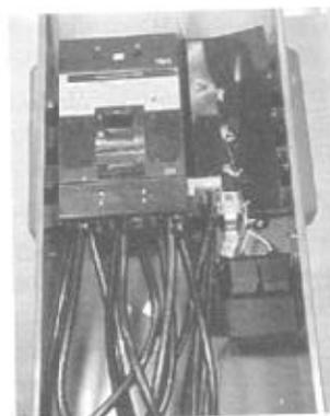
**Fig. 17-8** A surge (lightning) arrester installed in a service switch cabinet. Be sure its white wire is connected to the grounded neutral busbar in the cabinet. Take care to terminate its wiring at appropriate terminals; most main circuit breaker lugs are not listed for the combination of the small wires from the arrester and the much larger feeder or service conductors. Consult with the panelboard manufacturer for availability of appropriate terminations for the surge arrester. (Square D)
